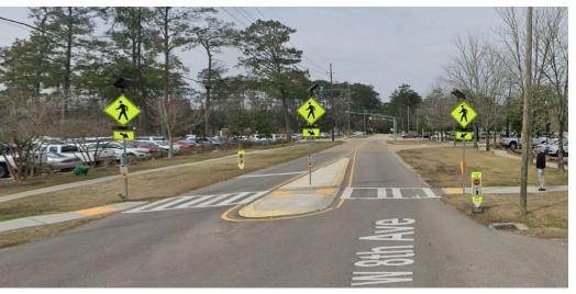
Rectangular Rapid Flashing Beacon assembly, known as the RRFB, is pedestrian actuated crosswalk beacon that flashes to alert drivers when someone is crossing. Shown here at W. 8<sup>th</sup> Ave in Covington.
